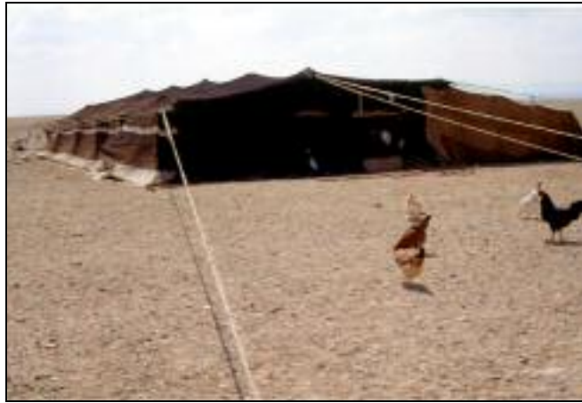
Fig. 1. A tent in Syria, near Palmyra, showing traditional construction using tensioning ropes. 1992.
