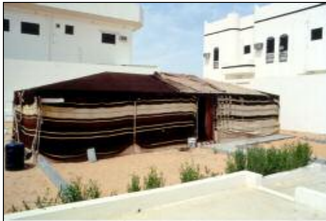
Fig. 8. Guest tent in a small yard. Because of lack of space, tensioning ropes were substituted with interior metal supports on a concrete base. Oneiza, central Saudi Arabia. 1992.
